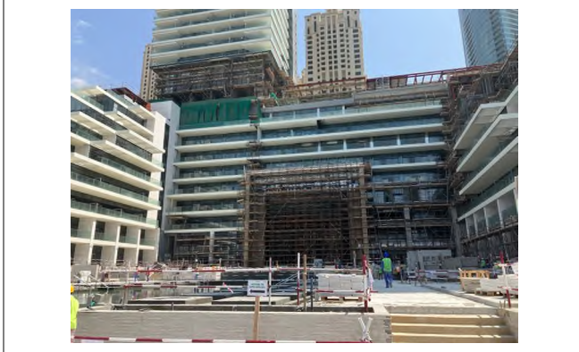
Source: CBRE Site Inspection
