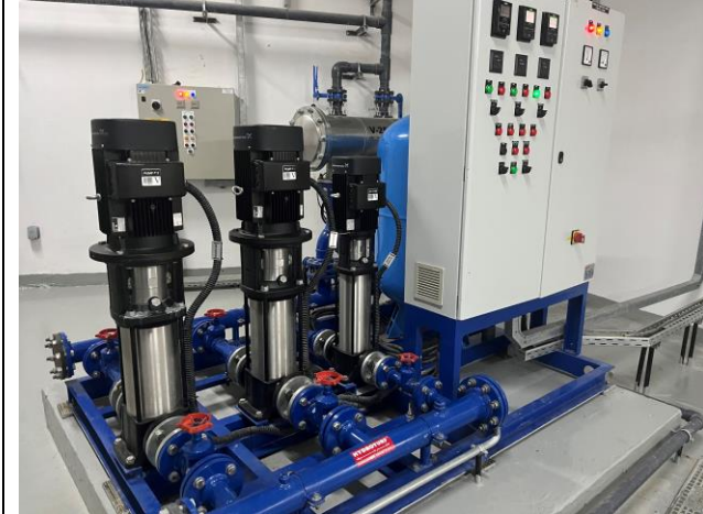
Irrigation water booster pumps in place (top) and site of future water pump (bottom) for distributing greywater to apartments landscaping.
