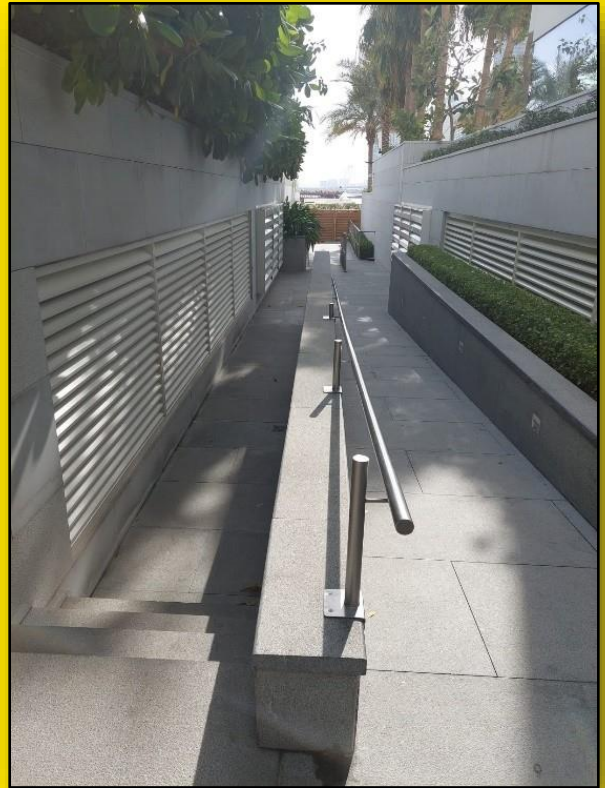
Ramps for mobility across premises for disabled and handicapped occupants
