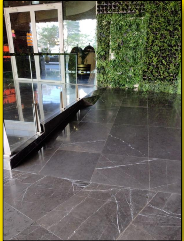
Disabled accessible ramps for building movement and entrance
